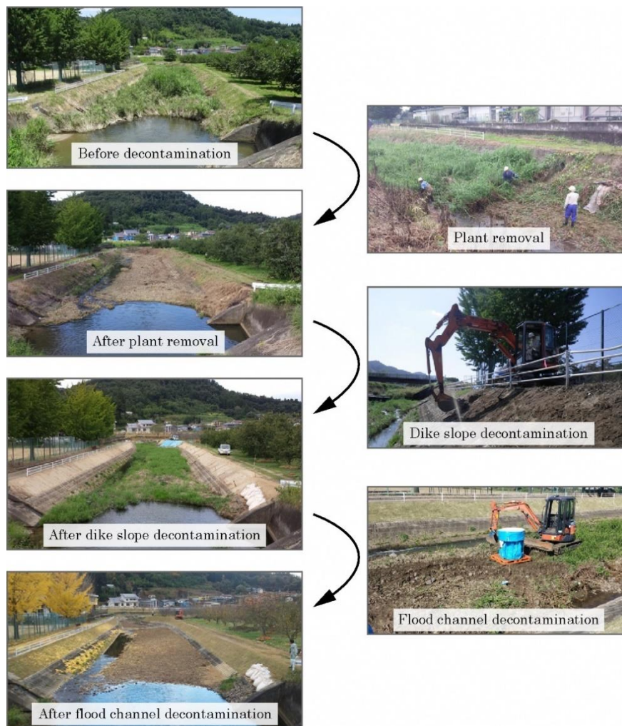
Figure 2. Photographs of the decontamination test procedures
